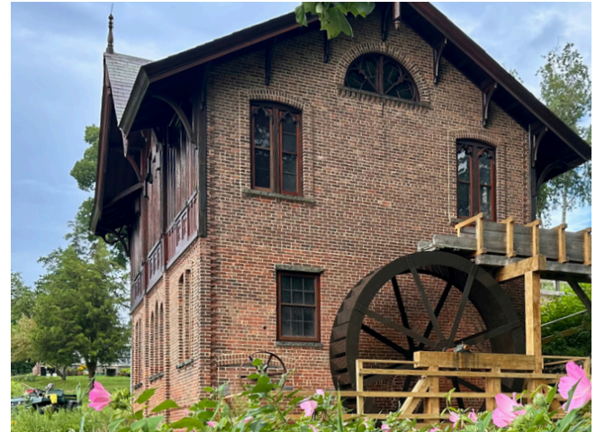
Keeping history alive: the Mill at Cedarmere is back in action after a meticulous restoration project. Photo: Tom Powell
